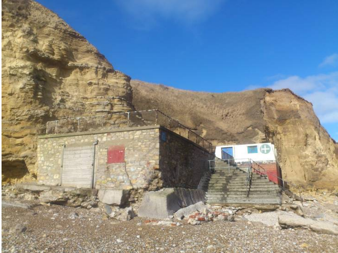
Plate 7 – Survey photograph 1bSS14_20130311_N4.jpg
