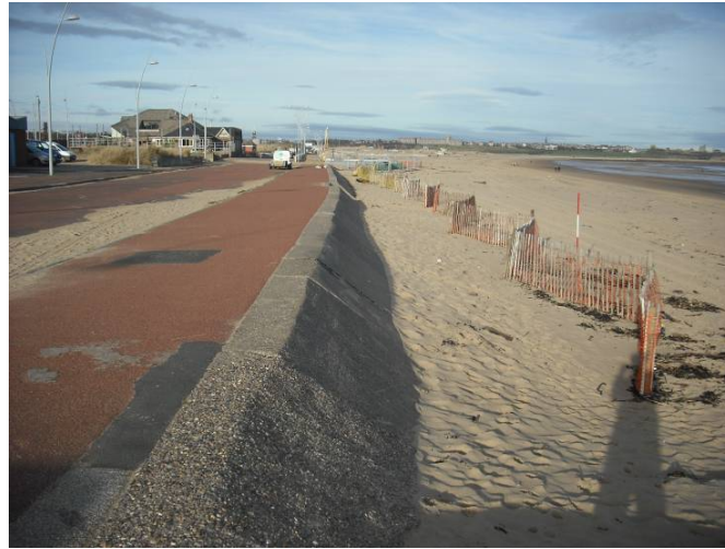
Plate 6 – Survey photograph 1bSS8_20121114_N1.JPG
