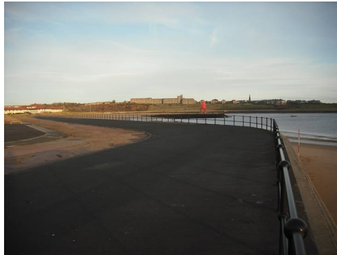
Plate 2 – Survey photograph 1bSS3_20121114_N2.JPG
