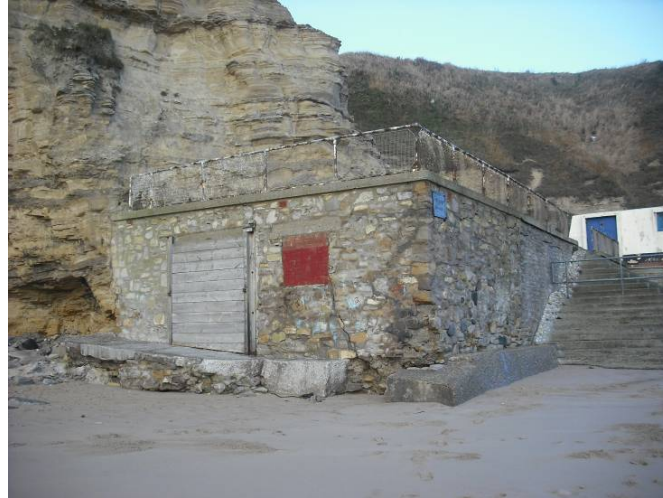
Plate 8 – Survey photograph 1bSS14_20121112_N2.JPG
