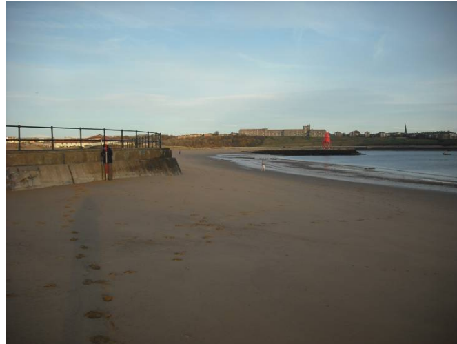
Plate 4 – Survey photograph 1bSS3_20121114_N3.JPG
