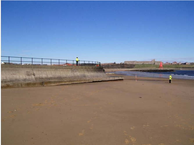
Plate 3 – Survey photograph 1bSS3_20130312_N3.JPG
